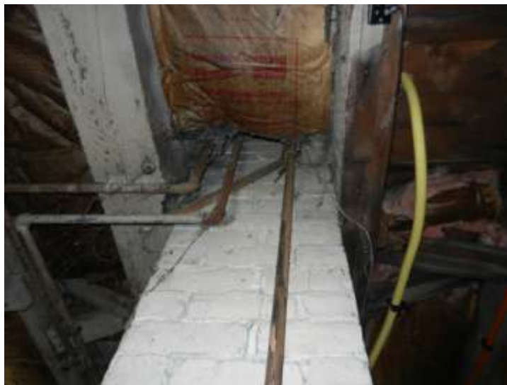
Basement chimney penetrations to attic need air sealing
