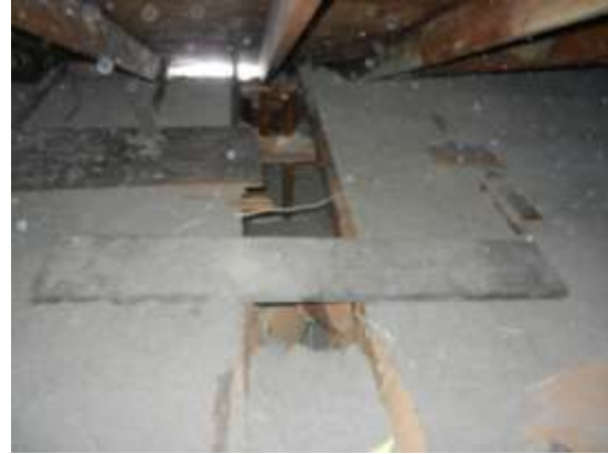
Large opening #2 in attic floor
