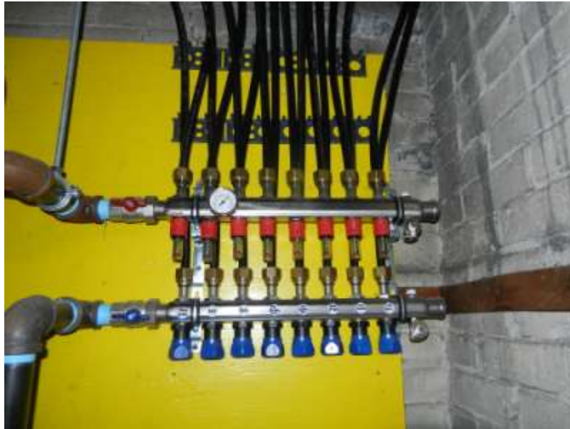
8 sets of return/supply ½" Pex Piping to Apt. #2
