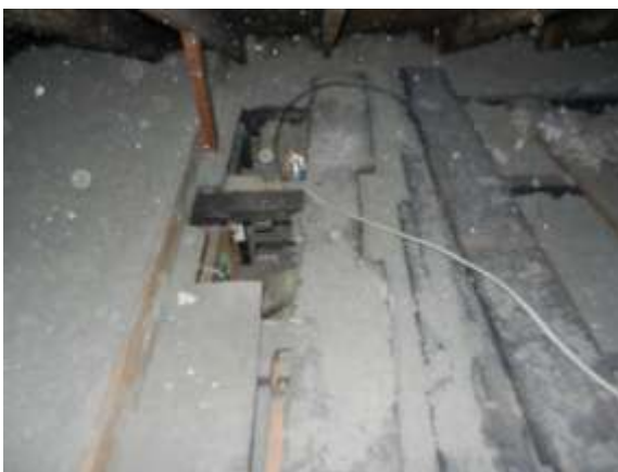
Large opening #1 in attic floor
