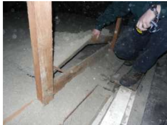
Less than two inch thick insulation on cardboard filler
