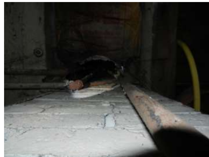
Basement chimney penetrations to attic need air sealing
