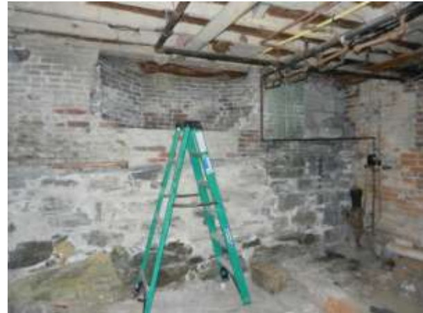
Field stone and brick foundation
