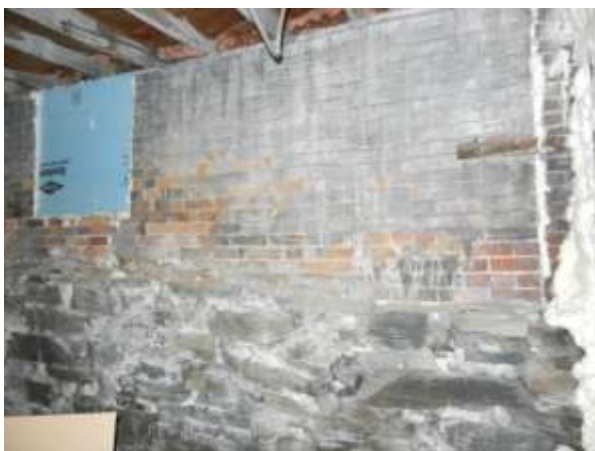
Field stone and brick foundation
