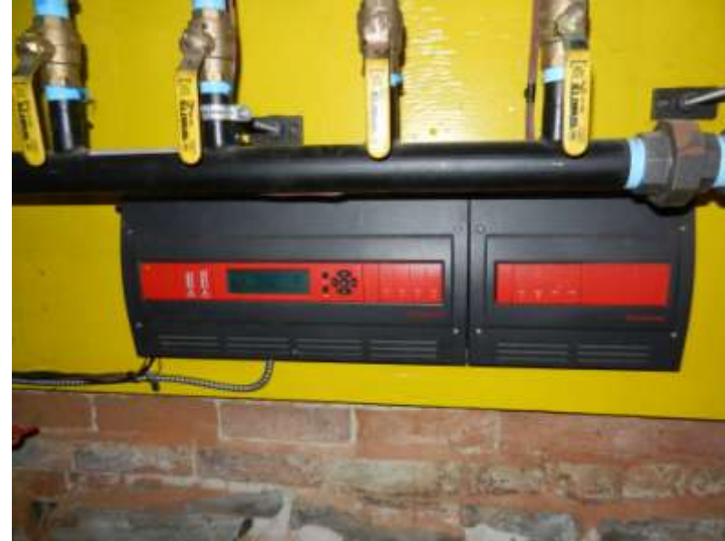
Honeywell outdoor reset controller
