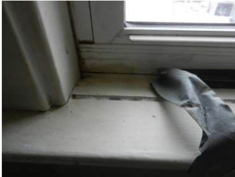
Typical interior window frame needs caulking to reduce infiltration
