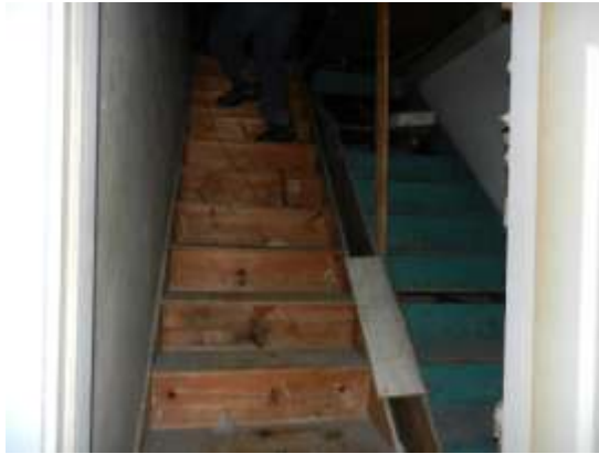
Double stairwell opening to attic
